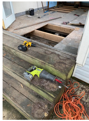
Rotting floor replaced in one of the dorms
