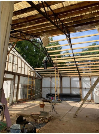
Atrium Roof Totally removed and replaced
