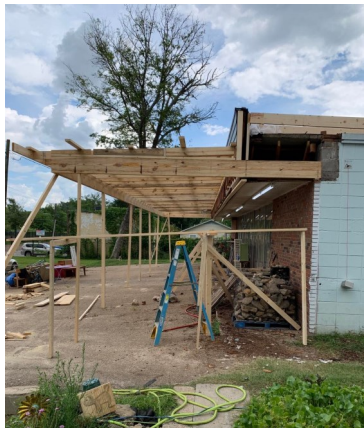
Clothes Closet got a new roof & a porch for more space!
