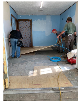
Rotting floor replaced in one of the dorms
